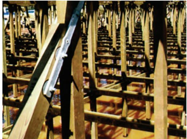
Transverse fan deck and hot water basin girts are 2" x 6"—all other transverse girts and all longitudinal girts are 2" x 4" except where loading may require 3" x 4". Transverse and longitudinal girts are spaced on 6'-0" vertical centers. Girt lines are through bolted to the columns.
